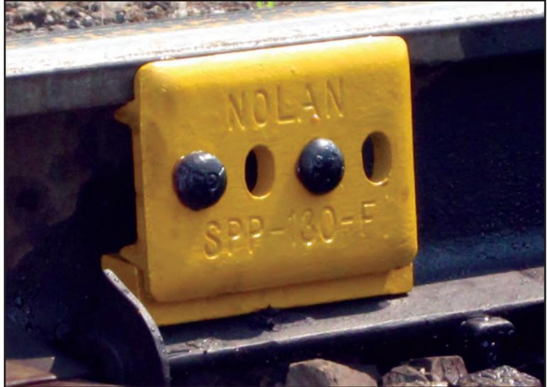
▲ SPP-6 installed on track with shim beneath
