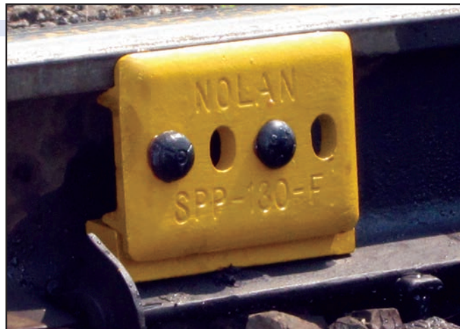
▲ SPP-6 installed on track with shim beneath
